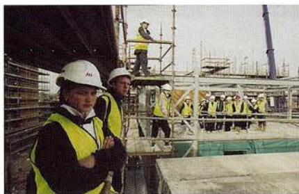
On site! Pupils from St Roch's, Royston, and Lochend Community High School, Easterhouse visit a 'live' construction site in Glasgow
